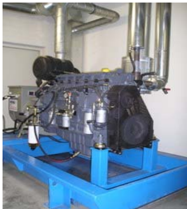
VWP Deutz DI engine for Jatropa oil
